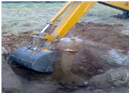
Fig.1. Removal of stub using JCB At Coimbatore
