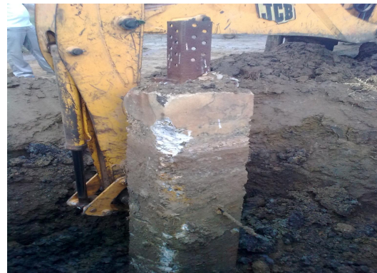
Fig.2 .Removal of stub using JCB at Chennai
