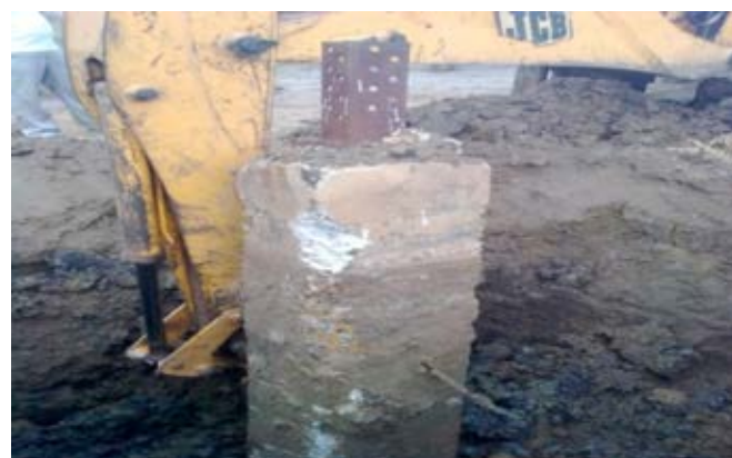
Fig.5. Removal of coastal stub
