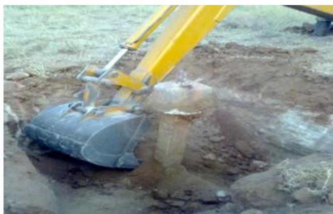
Fig.4. Removal of inland stub
