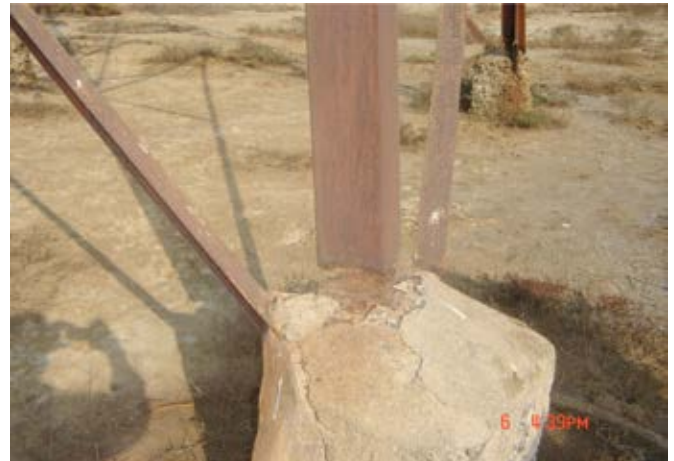
Fig.3. Snapping of stub angle
