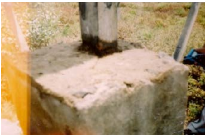
Fig.1. Formation of pitting corrosion at the angle concrete interface
