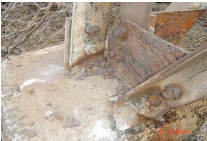
Fig.2. Bulging of stub angle
