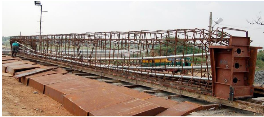
Fig. 1 Road bridge girder - skeleton reinforcement and sheathing pipes
