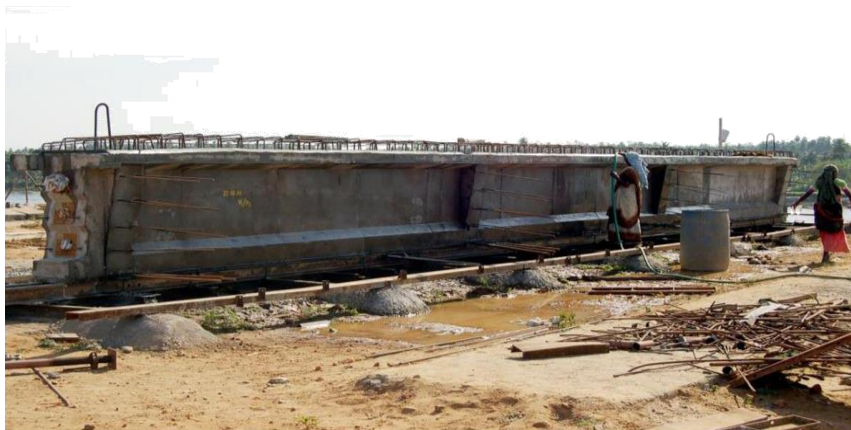
Fig. 2 Road bridge girder - after casting
