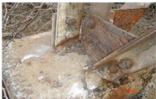
Fig 2. Ring of Rust at Interface of transmission tower stub at ground level
