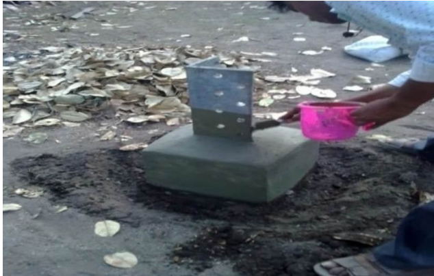
Fig. 9 — Flexibond coating on galvanized stub angle
