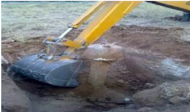
Fig. 10 — Removal of stub in Coimbatore (Inland)
