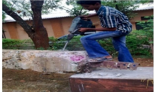
Fig. 12 — Stub excavated in Coimbatore (Inland)
