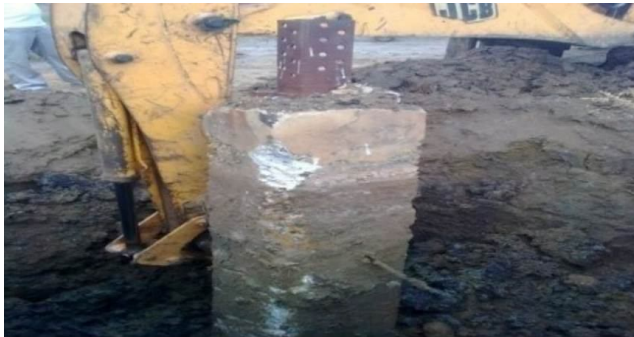
Fig. 11 — Removal of stub in Chennai (Coastal)
